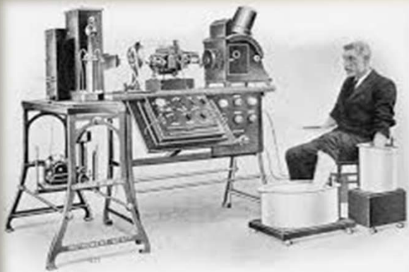
PHOTOGRAPH OF A COMPLETE ELECTROCARDIOGRAPH, SHOWING THE MANNER IN WHICH THE ELECTRODES ARE ATTACHED TO THE PATIENT. IN THIS CASE THE ELECTRODES WERE PLACED ON THE FOREARMS OF THE PATIENT.
